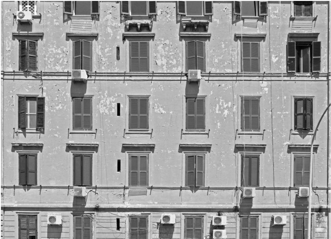
Fig. 1 - Historical, dense, worm, energy hungry, EU cities are facing several challenges for energy transition (Source: Fabrizio D'Angelo, 2023)
